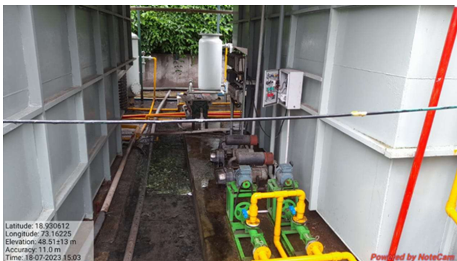
Figure 9.11.5 wastewater Treatment Plant
